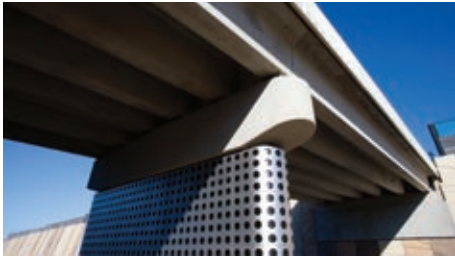
All EastLink's 88 bridges are clad with this unique design of stainless steel, which was manufactured by New Touch Laser Cutting in Bayswater.
